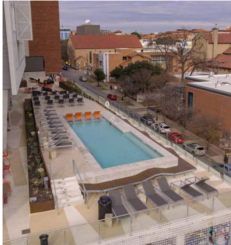
The University of Texas - SA Housing, Austin, Texas. Bone White and Franciscan Tan Classic Texture Contractor: Sundek of Austin
